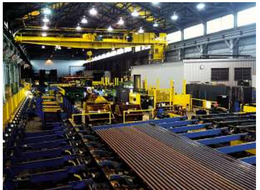
GGT supported the decommissioning, reinstallation and refurbishment works.
