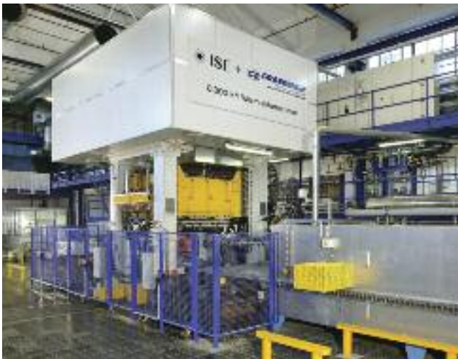
Evident in this photo of a Graebner hot-stamping line is the plumbing system on the back wall, for the line's chiller.
